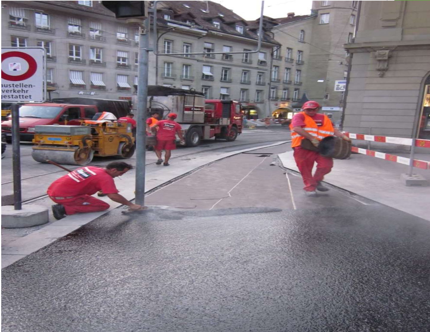
Sidewalk mastic asphalt paving Bern
