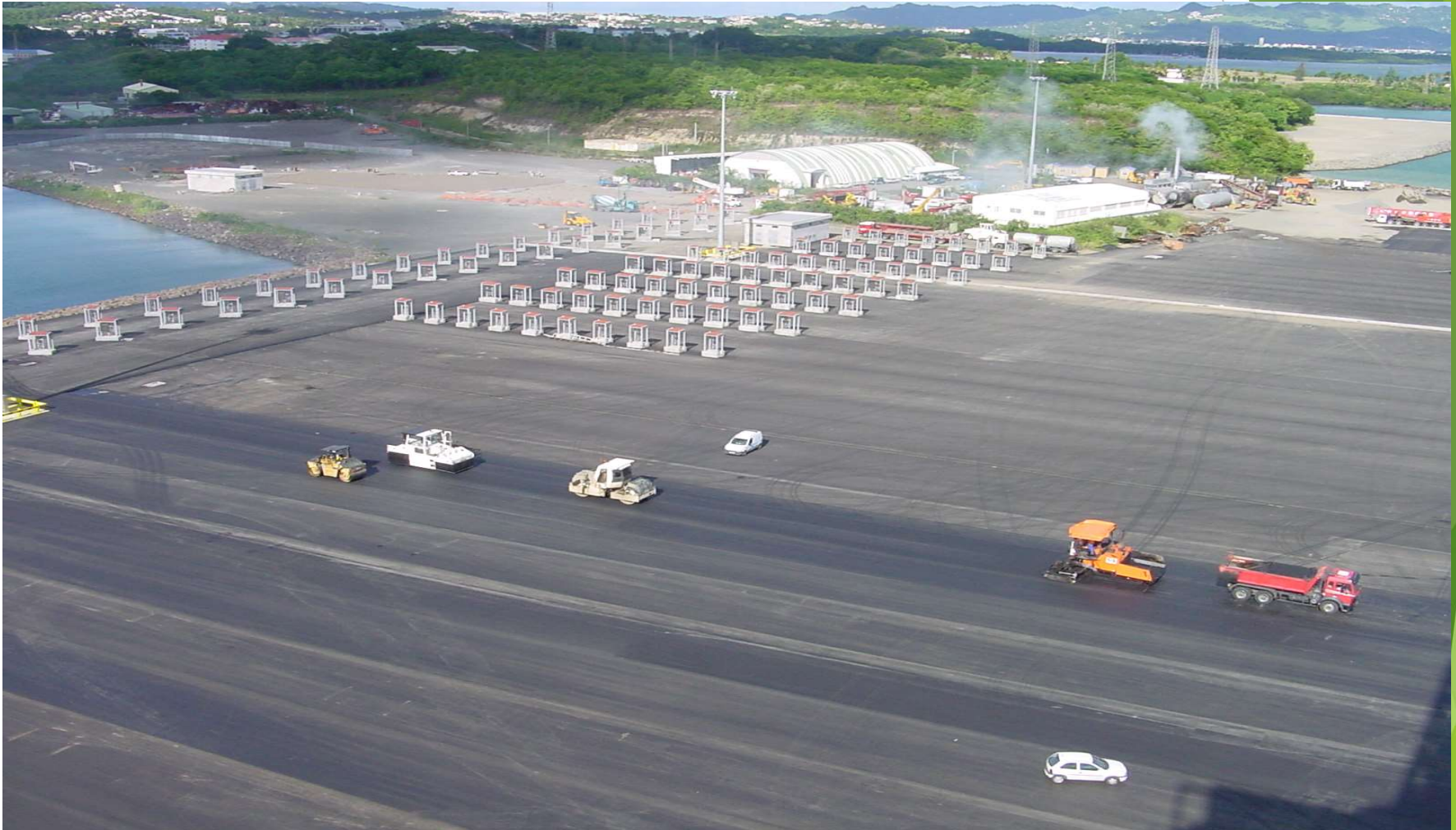
Port platform (France)
