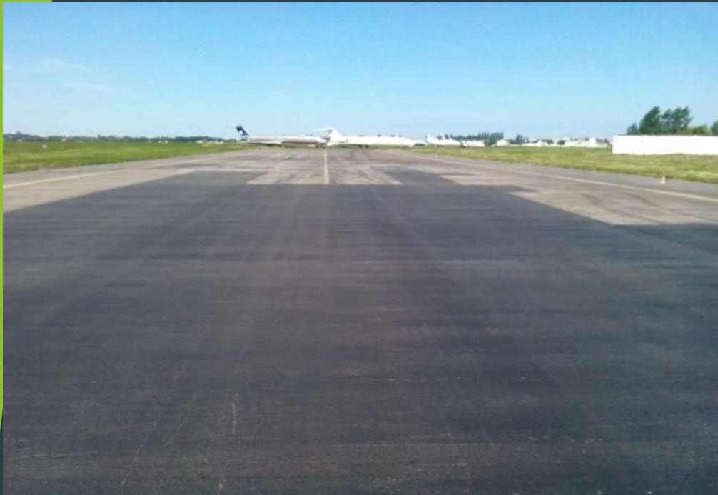
Works in Kiev International Airport (Zhuliany)
