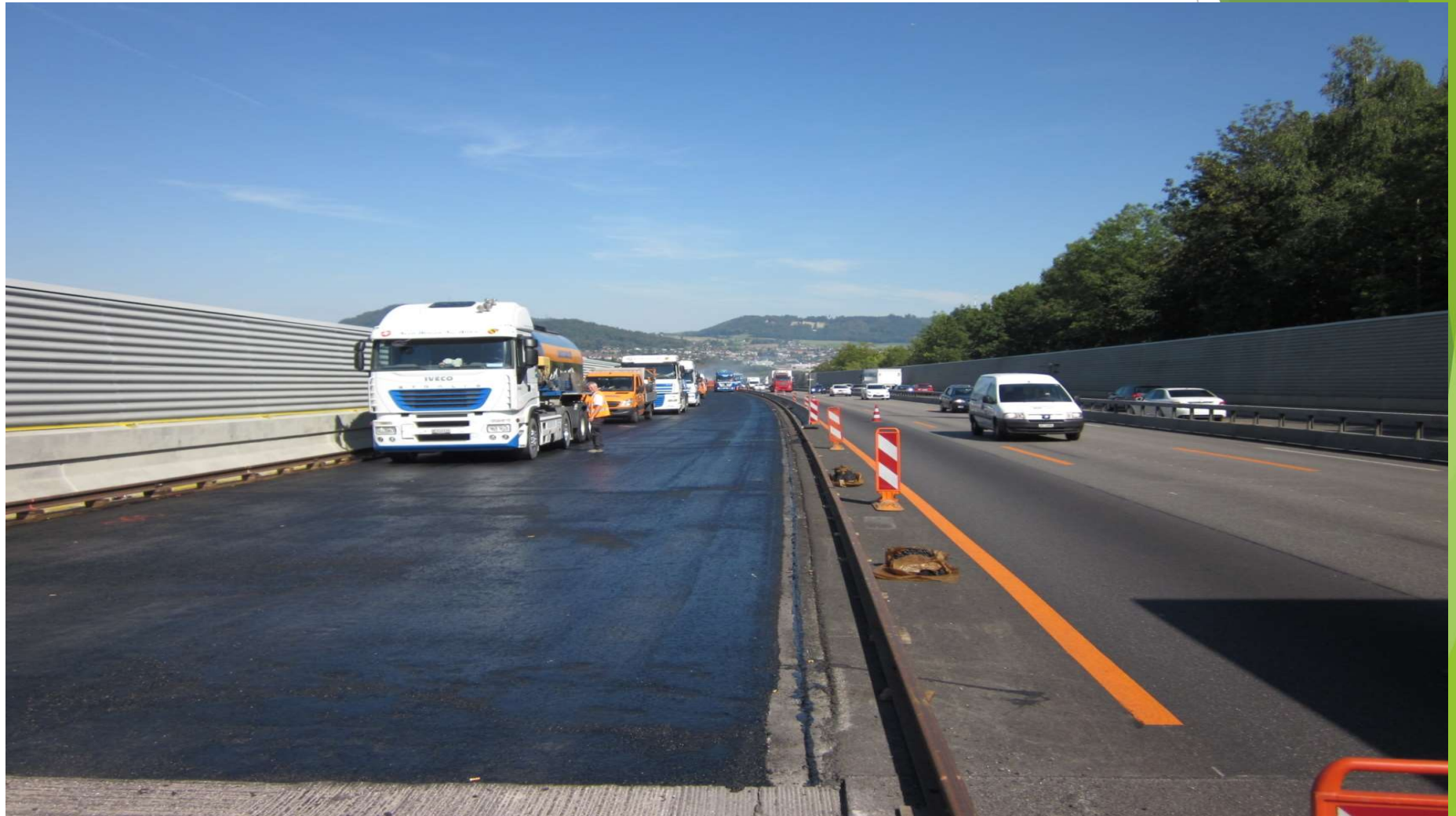
Mastic asphalt Bern
