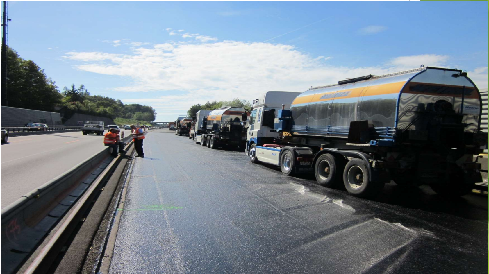
Mastic asphalt Bern
