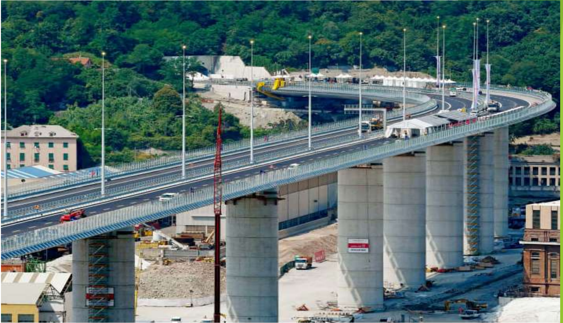
2020 New Genoa Bridge
