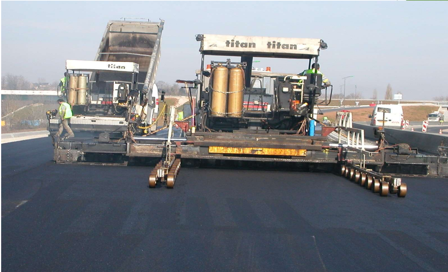
Road junction (France)
